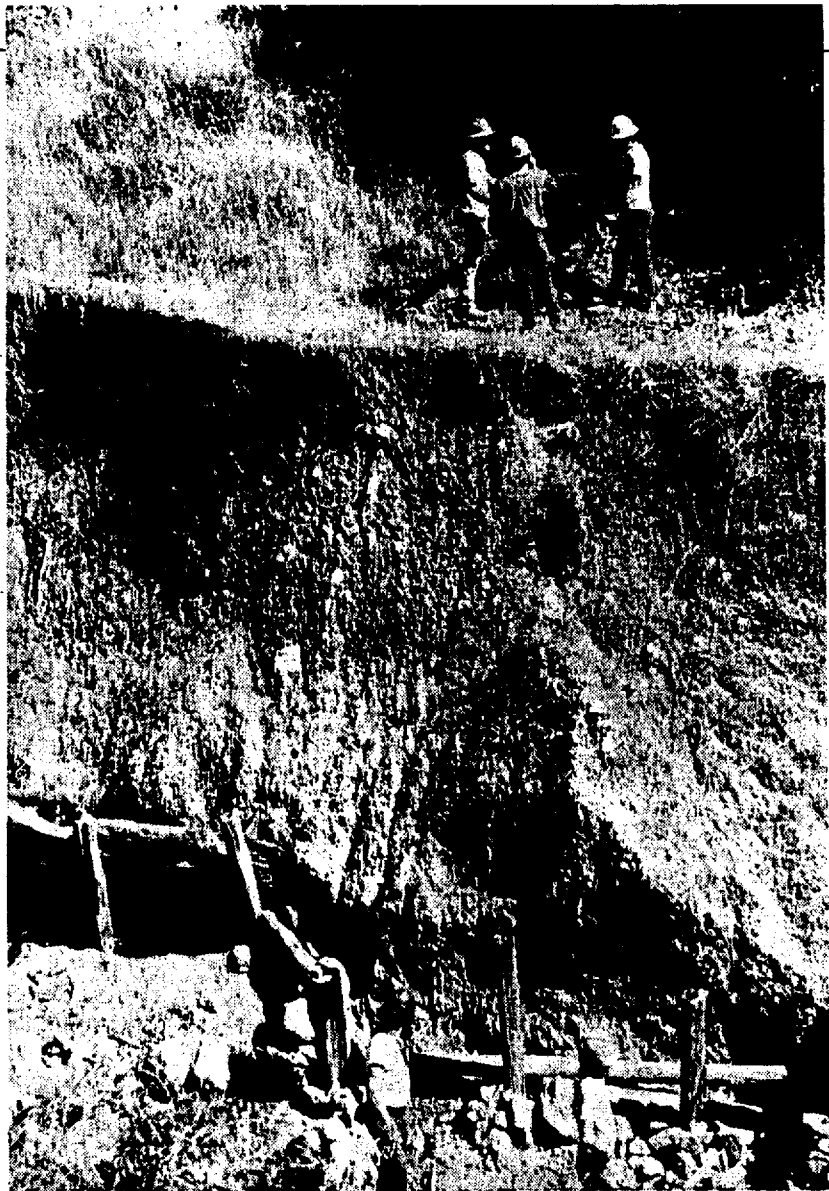
Cazadero Forest Workers' crew stabilizing the toe of a cutbank to prevent further erosion. Materials used came from a nearby log jam.
