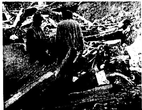
The author consults with old-timer Jimmy Kennedy about removing a log jam on Palmer Creek in the Gualala River watershed in Northern California. Some log jams act as barriers to spawning salmon. This one took a crew of eight one week to remove with hand tools.
